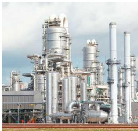
System expansion and post installation
